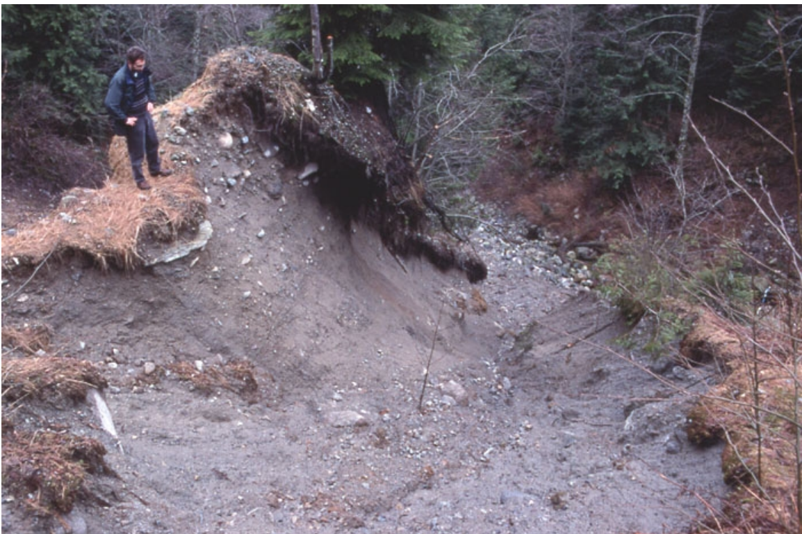
Photo 9 (above) and photo 10 (below). Photos looking downslope from road, showing deep erosion of fine silt slope material, on either side of remaining thin, erect island of material where person is standing. Note that the island is supported by tree roots. This island will let loose at any time, as slope is continuing to erode, and has considerably weakened as a support for the road directly above. Hurricane Creek is directly below, where washed silts from slide material, causes turbidity, and is transported directly into Capilano Reservoir.
