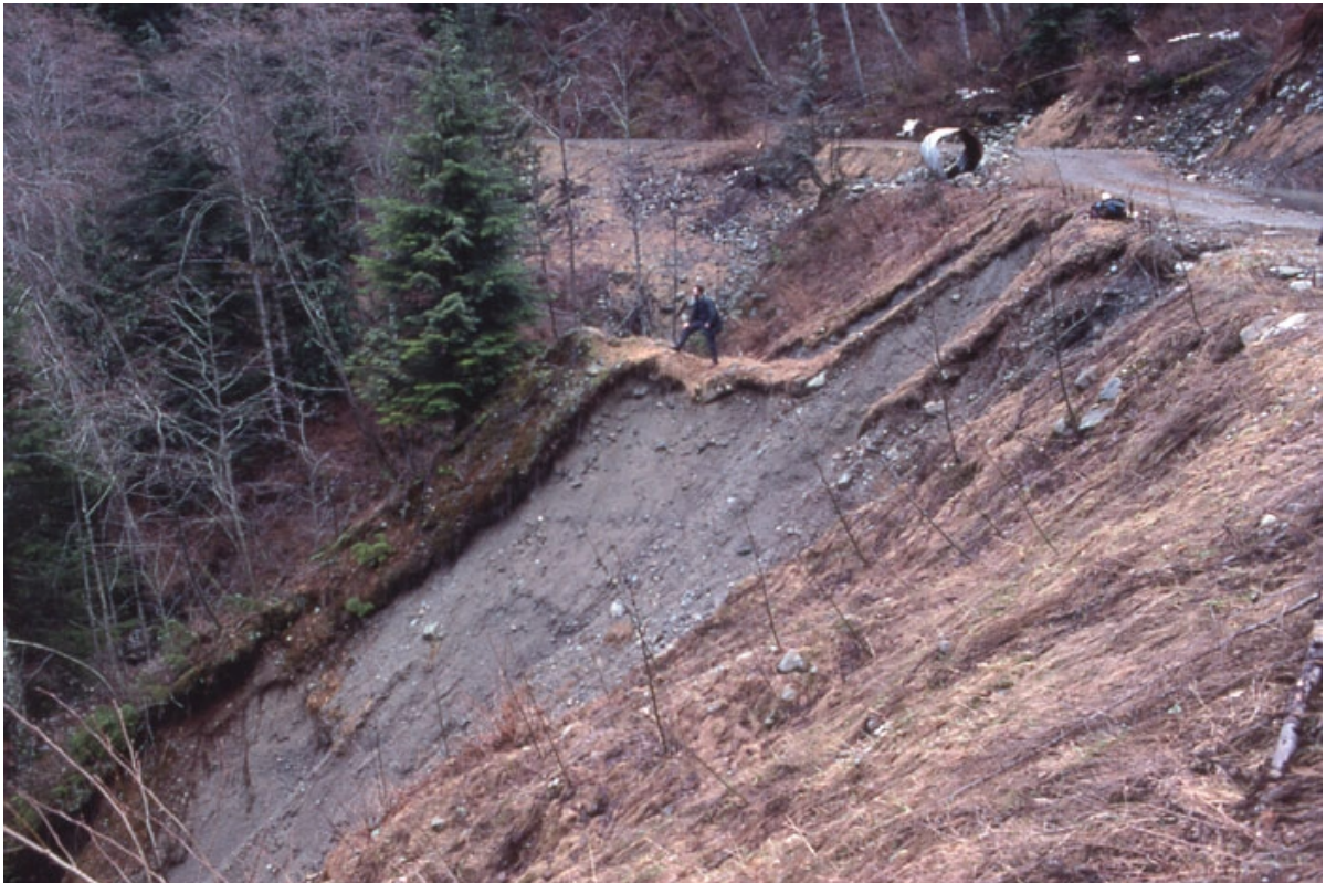
Photo 8 (below). Reverse angle of photo 7, showing large slope failure below road. Note person in middle of photo for scale. Hurricane Creek is about 100 feet behind person.
