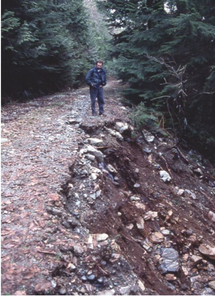
Photo 3 (left). Directly to left of person standing is the point where the diverted water runoff went down the slope, supersaturating the soil, and causing a small landslide.
