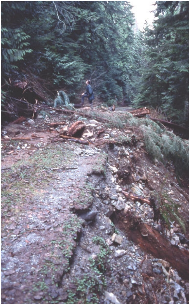
Photo 5 (above). Shows the upper landslide area from lower road. For scale, note person in upper middle area. Water runoff diverted to right and left of photo, and down road ditch to right.
