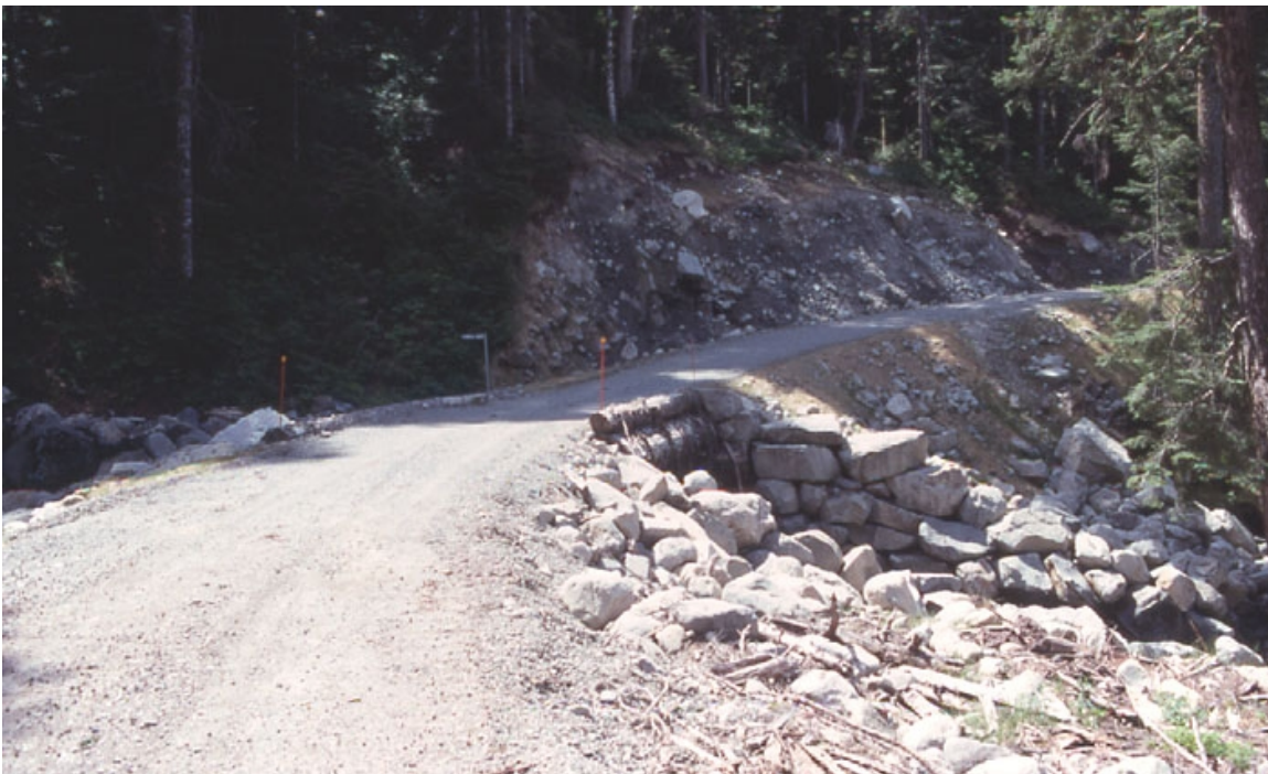
Another large cutslope at upper end of Eastcap logging road, next to Cypress Creek. Note person in upper photo, on logging road, for scale. These sediments are routinely washed into the Capilano River during heavy rainstorms. Photo below shows same area, but from another angle across Cypress Creek bridge.
