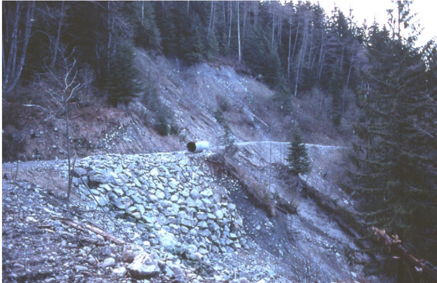
Photo 7 (left). Large top and bottom cutslopes in area 2 (see page 10), the source of fine silt erosion and turbidity.
