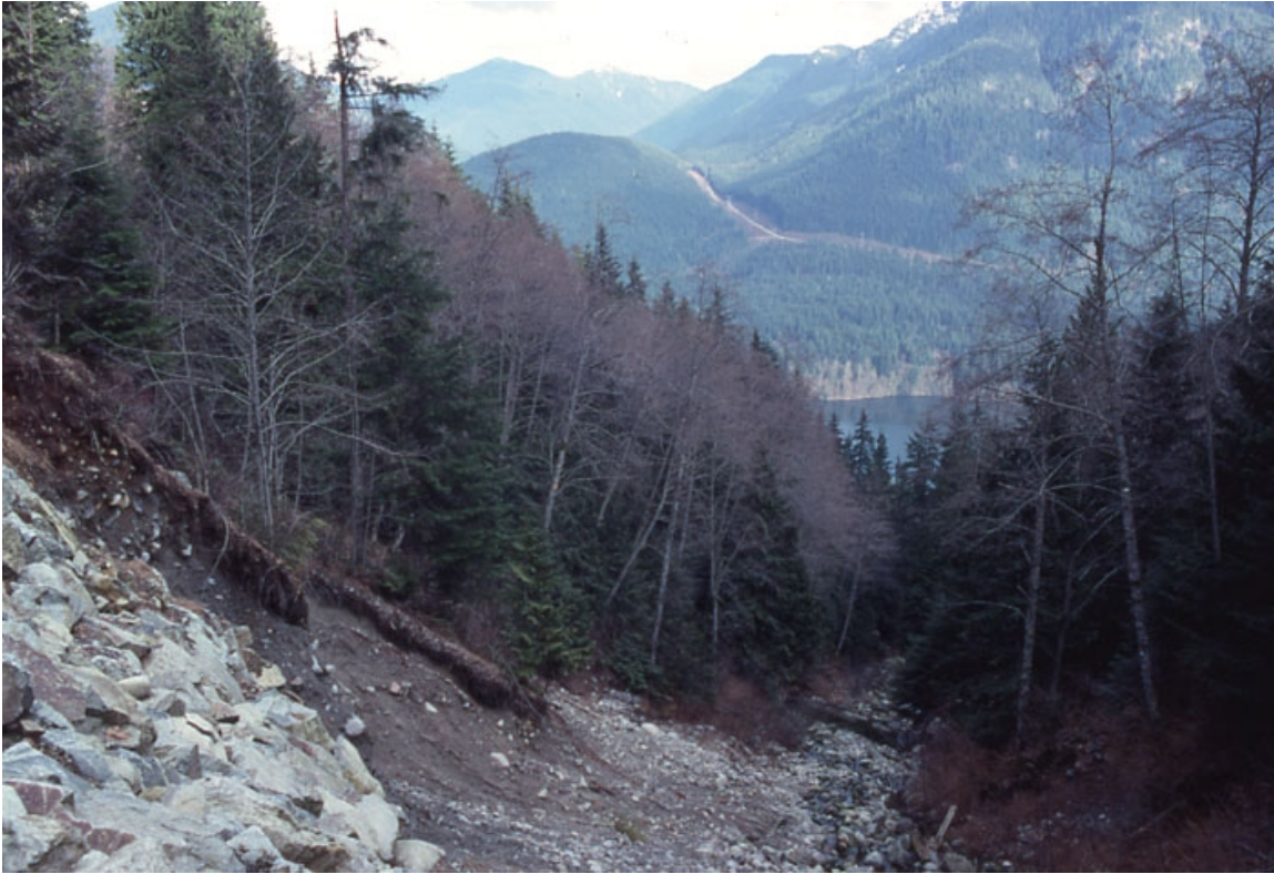
Photo 11. Looking down Hurricane Creek. Note Capilano Reservoir below. Note eroded banks to bottom left area. All debris washed into creek and down into reservoir. The Water District previously placed rip-rap (rock) on slope to support road and bank to bottom left..
