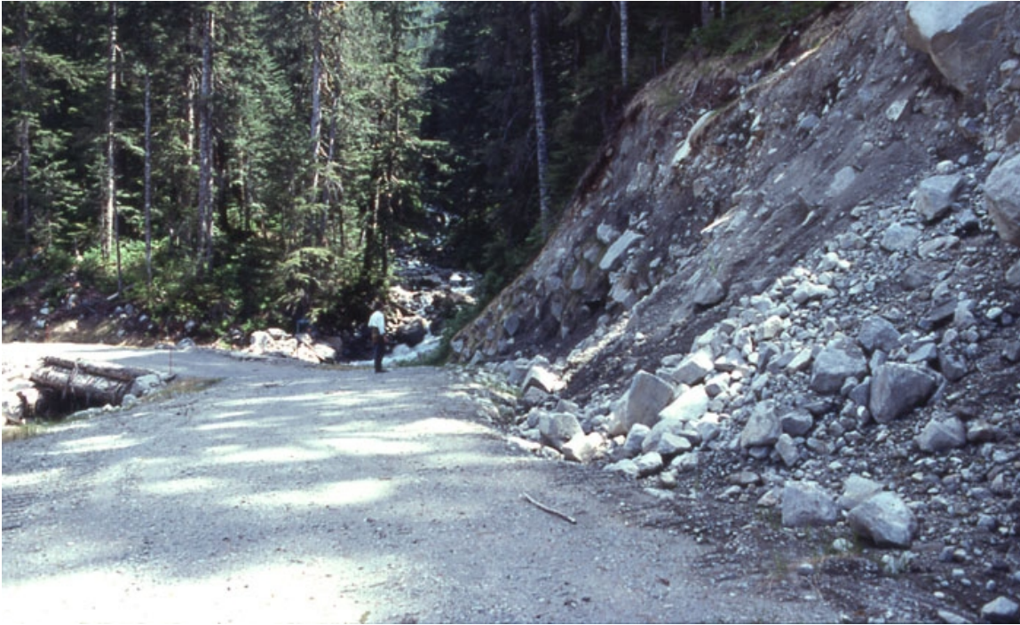
Another large cutslope at upper end of Eastcap logging road, next to Cypress Creek. Note person in upper photo, on logging road, for scale. These sediments are routinely washed into the Capilano River during heavy rainstorms. Photo below shows same area, but from another angle across Cypress Creek bridge.
