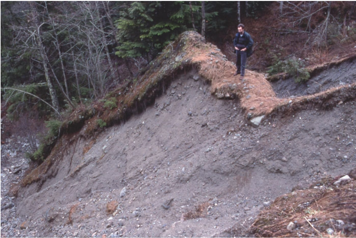
Photo 9 (above) and photo 10 (below). Photos looking downslope from road, showing deep erosion of fine silt slope material, on either side of remaining thin, erect island of material where person is standing. Note that the island is supported by tree roots. This island will let loose at any time, as slope is continuing to erode, and has considerably weakened as a support for the road directly above. Hurricane Creek is directly below, where washed silts from slide material, causes turbidity, and is transported directly into Capilano Reservoir.
