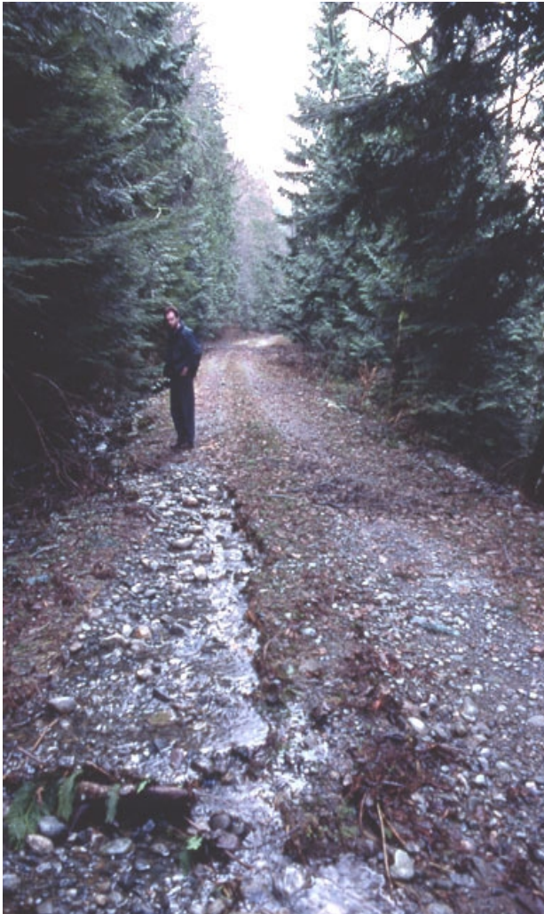
Photo 1 (left). Runoff water diverted onto road due to blockage in ditch. Road grade is about 20 percent.
