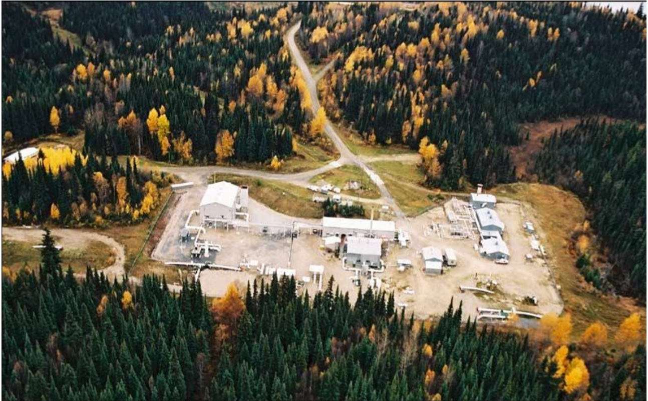
Photo of Summit Lake facility north of Prince George, the site of Pacific Northern Gas's current westward gas extension pipeline to Prince Rupert, and the site of the new proposed 36 inch diameter pipeline link to Kitimat.
