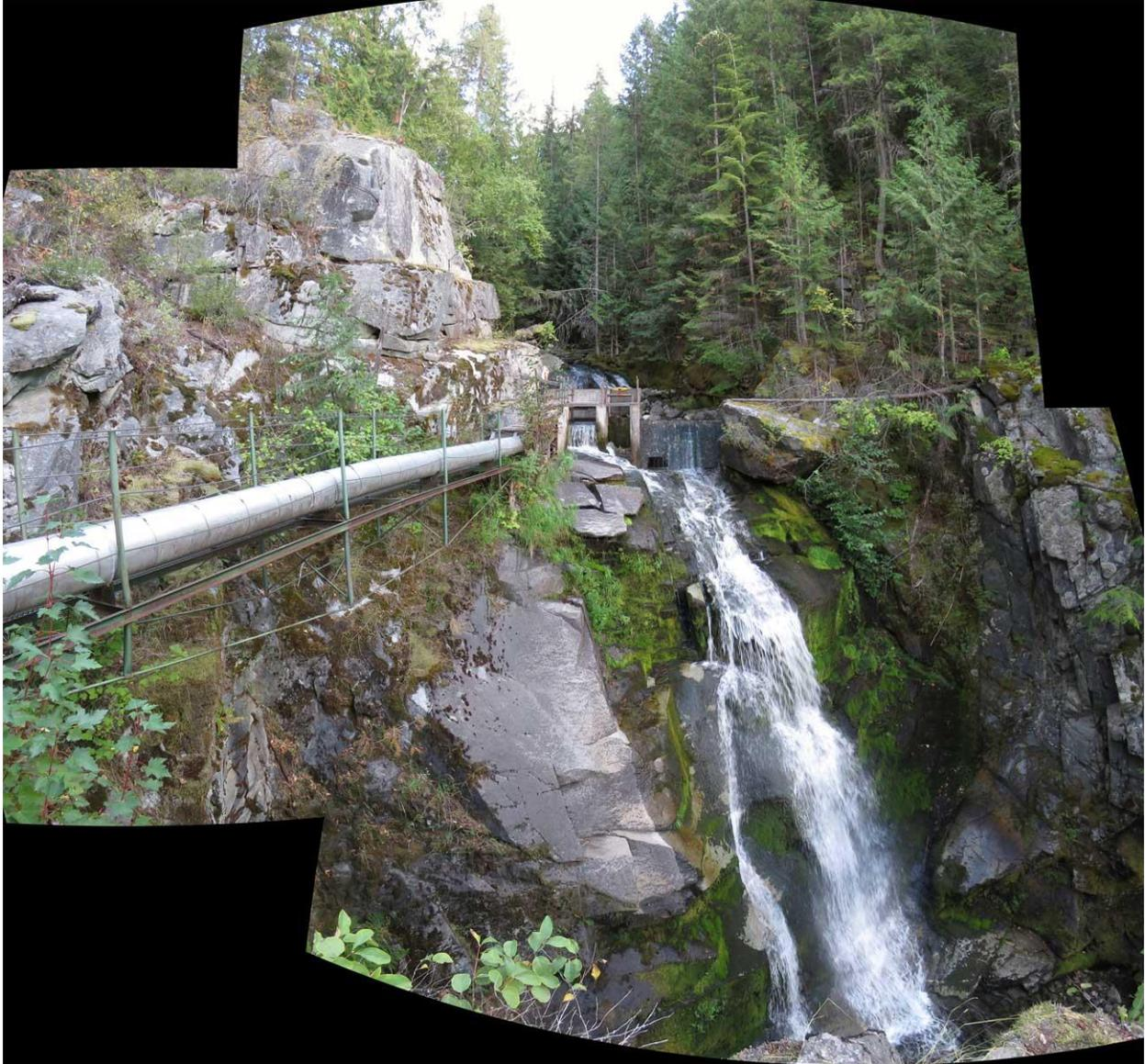
Photo collage of the Glade intake on Glade Creek (September 2016). The small concrete dam, located in a ravine, is nested just above a steep waterfall. The water pipeline and gangplank is constructed along the granite wall of the ravine, which leads to a control building nearby. Logging has the potential to destroy the intake facility.
