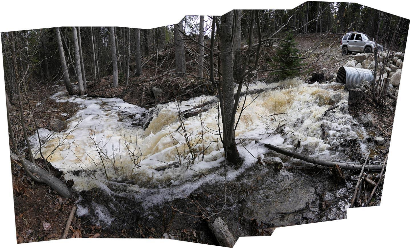
Photo stitch 70 (May 4, 2018). Just below Photo 69, a large culvert was recently placed under a forest access road. The heavy water runoff continues downslope, cutting through soils that were never eroded before, accustomed to only smaller flows.
