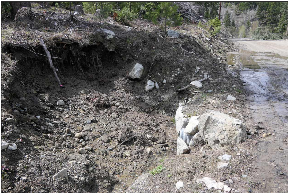
Photos 20 and 21 (April 30, 2018). Glacial silt muck oozing out of small cutslopes causing blockage of culvert and water runoff to spill across road prism and down ditches and ephemeral streams. About 4-kilometer mark.
