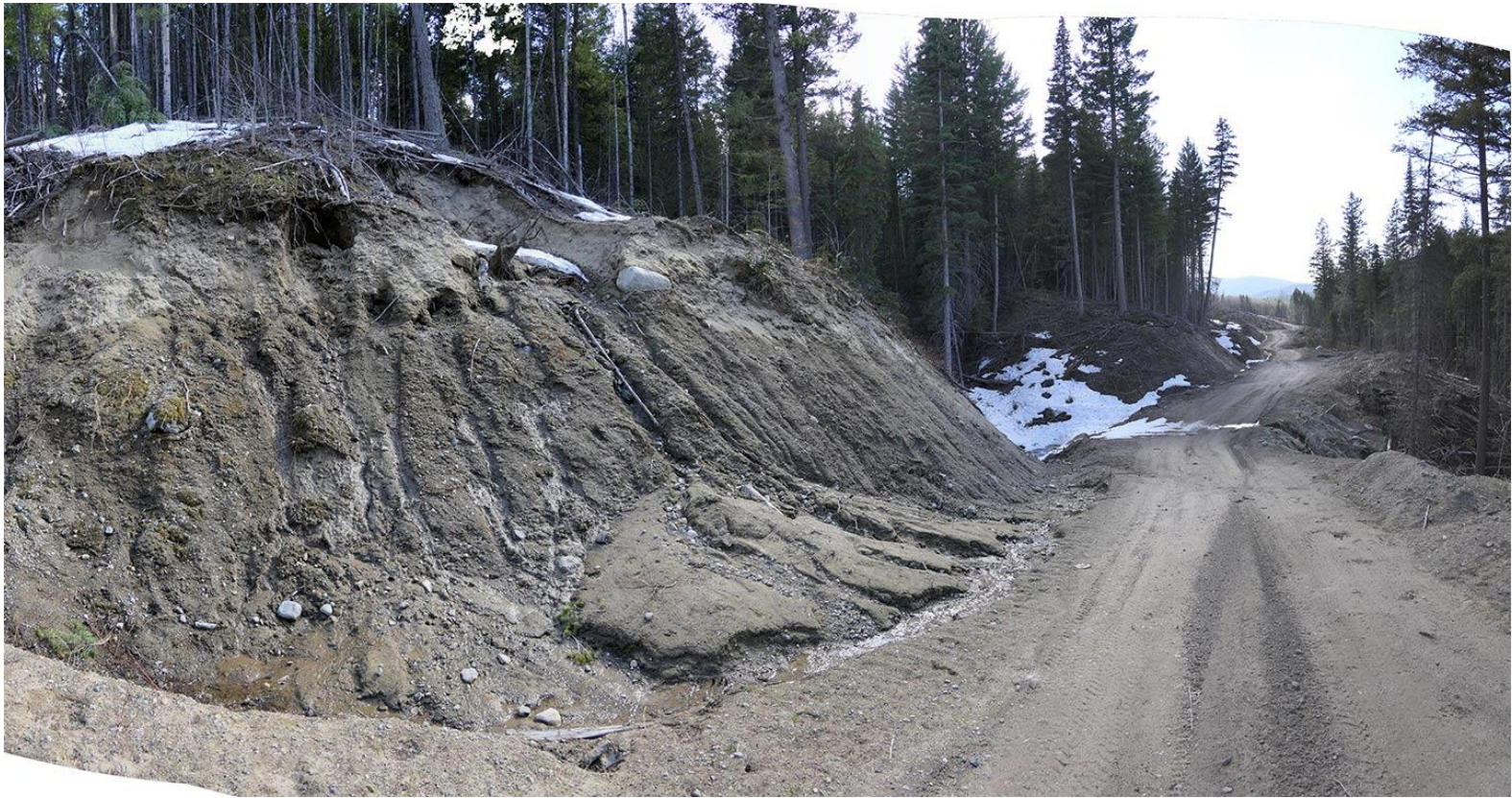
Photo stitches 36 and 37. Below, ditch water from cutslope was running strong, and eroded road prism above culvert.
