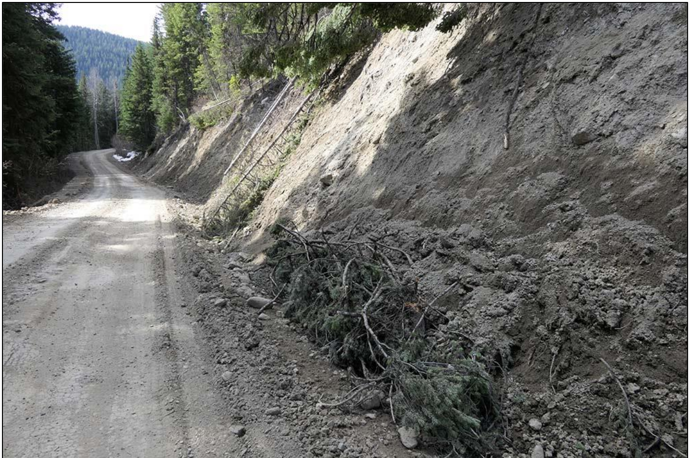
Photo stitches 46 and 47 (May 5, 2018). The Glen Lake forestry road bends around Bolivar Creek, a tributary to Greata Creek, just below the photos to the left. The road cuts through fine glacial lacustrine soils which are eroding off the road, and into the Creek below. There is no ditch along this section of the road, nor were any culverts placed (if so, they were hidden somewhere).
