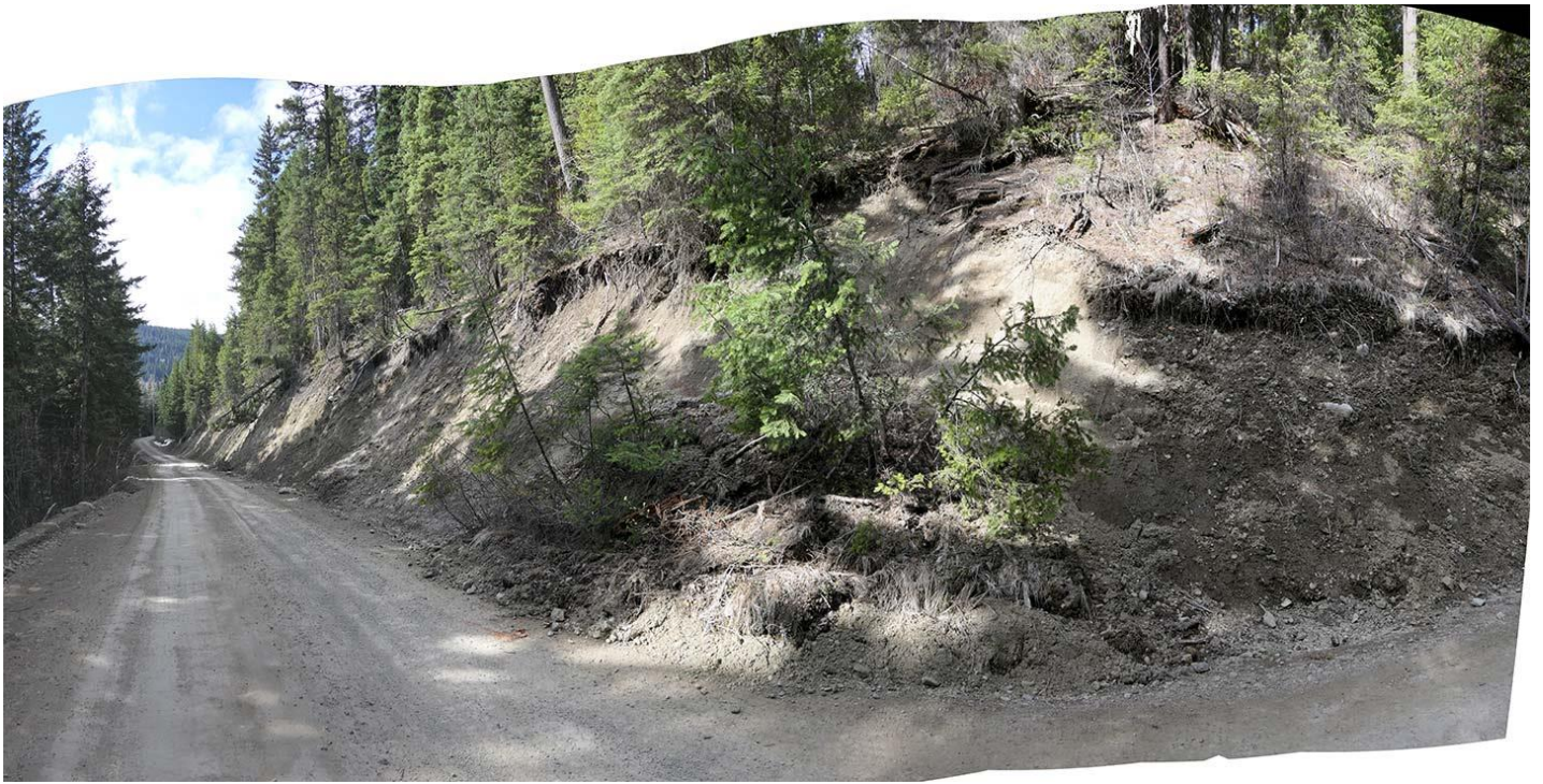
Photo stitches 46 and 47 (May 5, 2018). The Glen Lake forestry road bends around Bolivar Creek, a tributary to Greata Creek, just below the photos to the left. The road cuts through fine glacial lacustrine soils which are eroding off the road, and into the Creek below. There is no ditch along this section of the road, nor were any culverts placed (if so, they were hidden somewhere).
