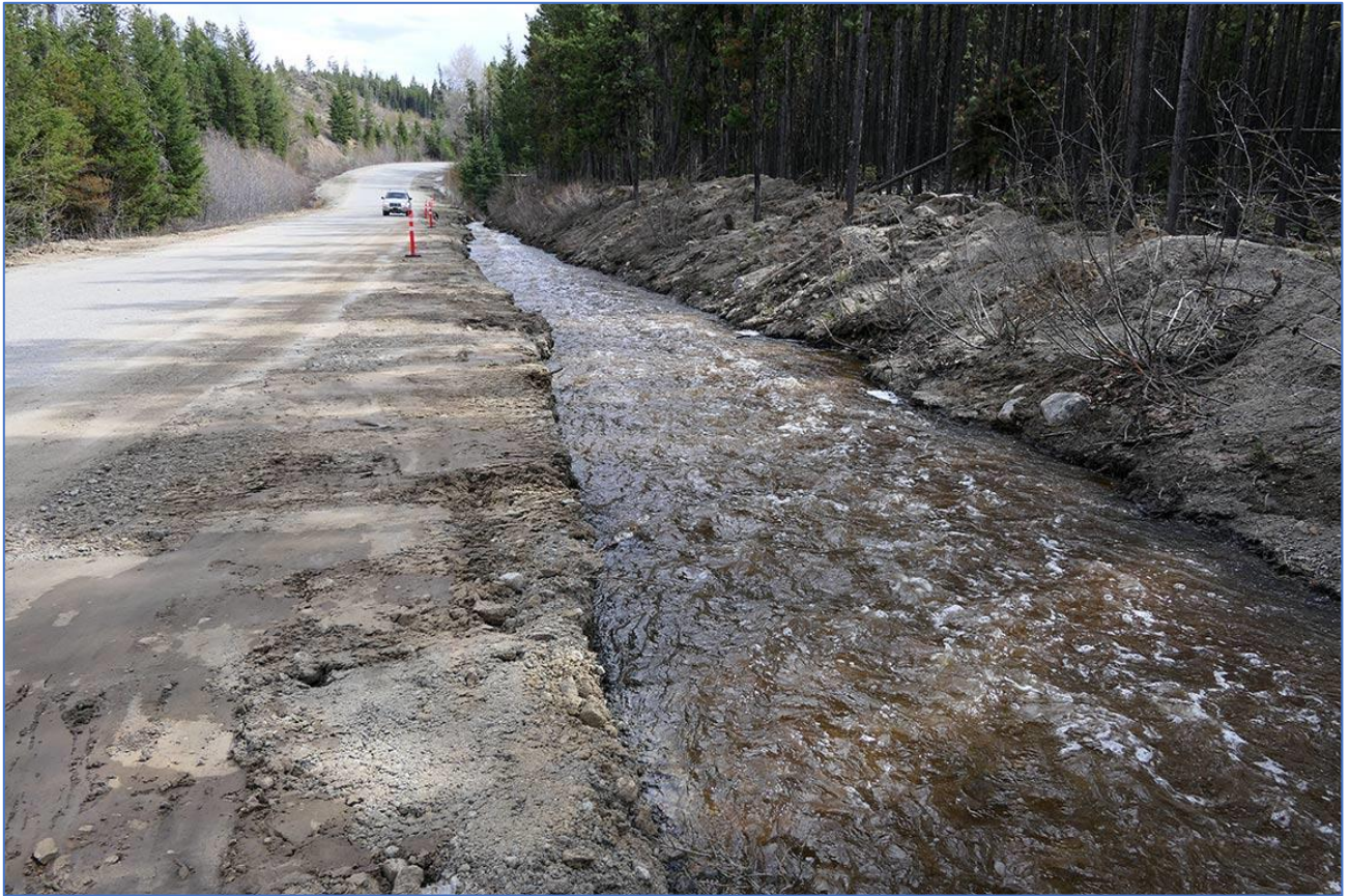
Photo 75 (May 4, 2018). 75 meters down from Photo 74 , the water is running high and turbid, despite the efforts to dig the newly scoured ditch deeper.
