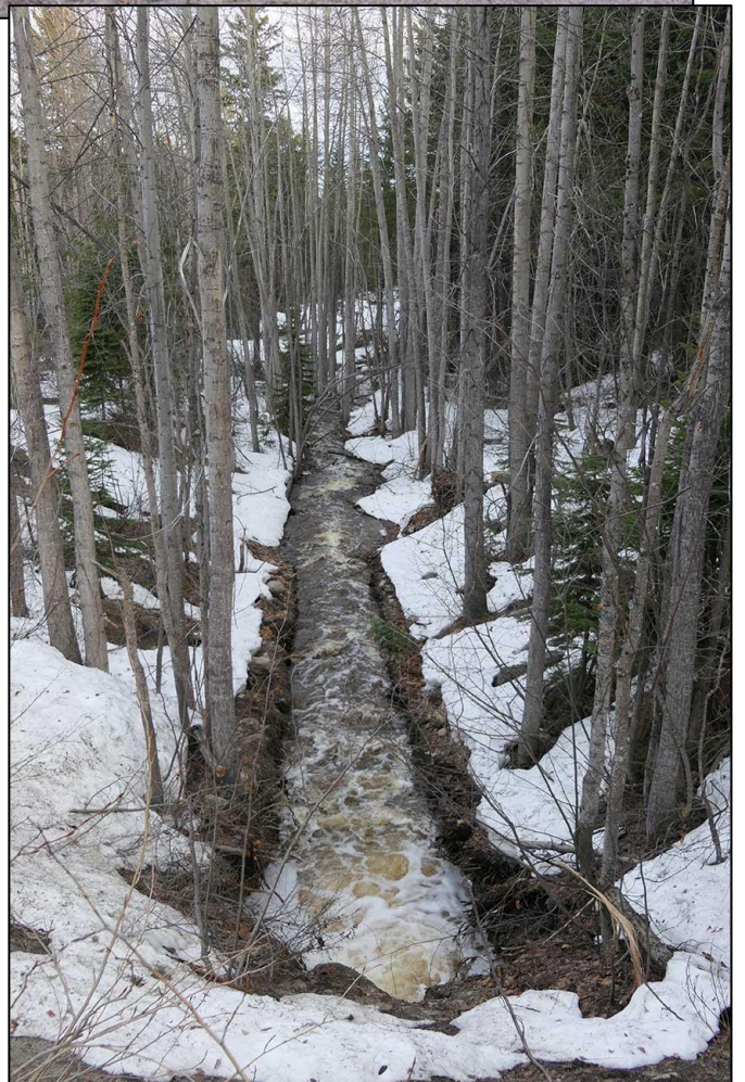
Photo 68 , above (April 30, 2018). Close up of area in Photo 67 . The water runoff was too much for the small culvert under the Princeton road in 2017, and no doubt due to some blockage, that the water quickly pooled in the area to left bottom of photo, and then spilled down the road ditch, eroding the ditch.
