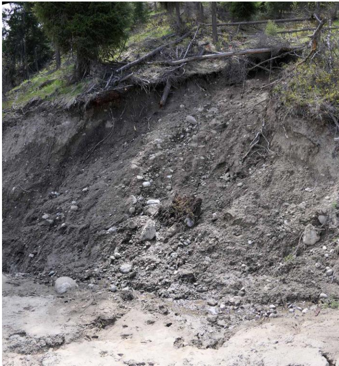
Photos 13 to 15 (April 30, 2018). Multiple scenes showing cutslope slumping and resulting culvert blockages, with culverts recently and partially cleared by maintenance crew.
