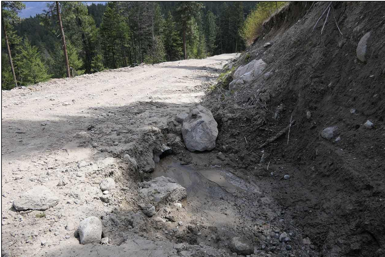
Photos 11 and 12 (April 30, 2018). From one to two kilometers above the Munro switchback, about 5 culverts were blocked by cutslope materials and debris. Cutslope slumping of fine glaciolacustrine silts and till were transported far down the road, which had little to no ditching, creating long, wide wash torrents during snow melt. Below, a culvert, recently and partially cleared by maintenance workers, still shows signs of blockage.
