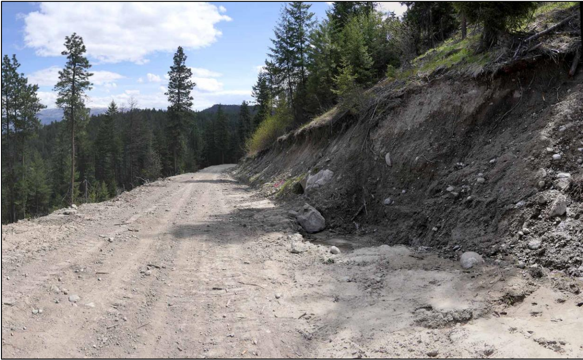
Photos 11 and 12 (April 30, 2018). From one to two kilometers above the Munro switchback, about 5 culverts were blocked by cutslope materials and debris. Cutslope slumping of fine glaciolacustrine silts and till were transported far down the road, which had little to no ditching, creating long, wide wash torrents during snow melt. Below, a culvert, recently and partially cleared by maintenance workers, still shows signs of blockage.
