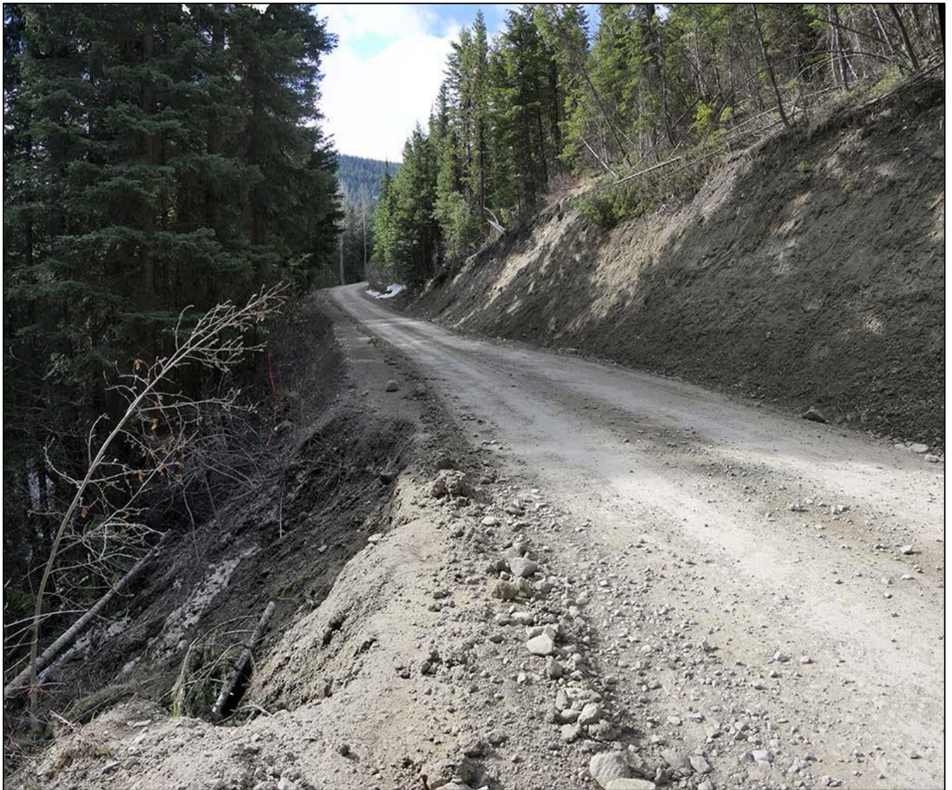
Photo stitch 48 (May 5, 2018). This is the same area as in photos 46 and 47, showing the collapse of a cutbank into Bolivar Creek. Water runoff pooled and poured across the road, causing this area to fail. Photo stitch 49, below (May 5, 2018). Greata Creek is running turbid, not clear.
