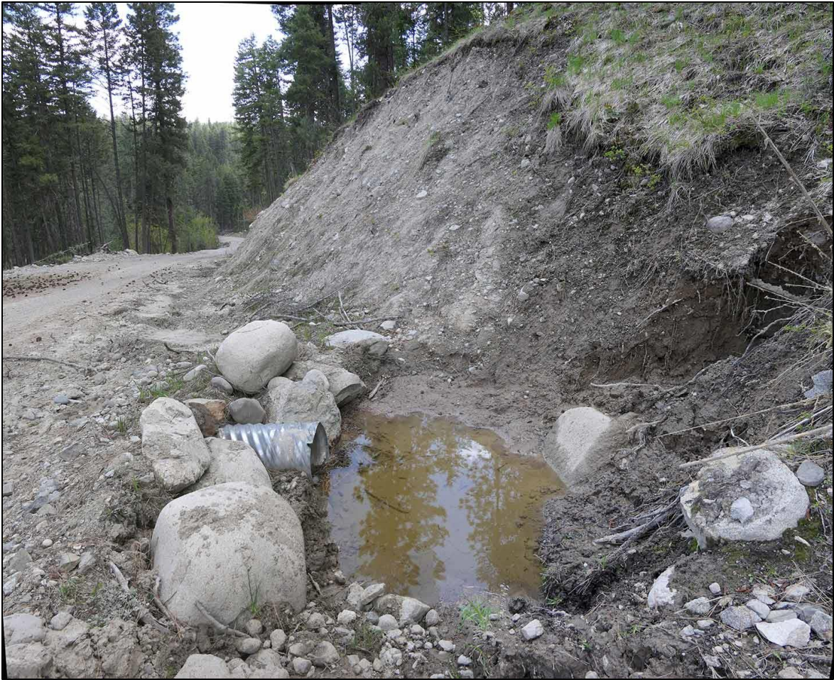
Photos 13 to 15 (April 30, 2018). Multiple scenes showing cutslope slumping and resulting culvert blockages, with culverts recently and partially cleared by maintenance crew.
