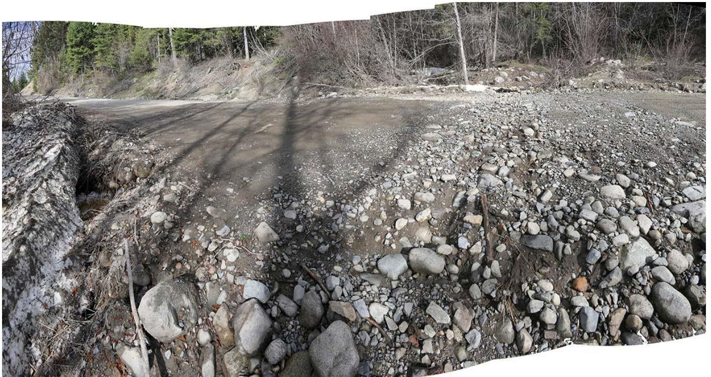
Photo stitches 44 and 45 (May 5, 2018). Small creek overflowing because the culvert is too small, and slightly plugged. Recent high water, and erosion of road prism.
