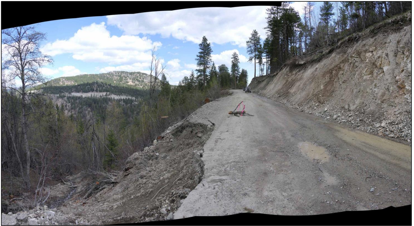
Photo stitch 16 and photo 17 (April 30, 2018). Road failure around the 3.5-kilometer mark on Munro Road. Debris has fallen into stream channel above Peachland Creek. The Princeton access road is seen in distance to left.
