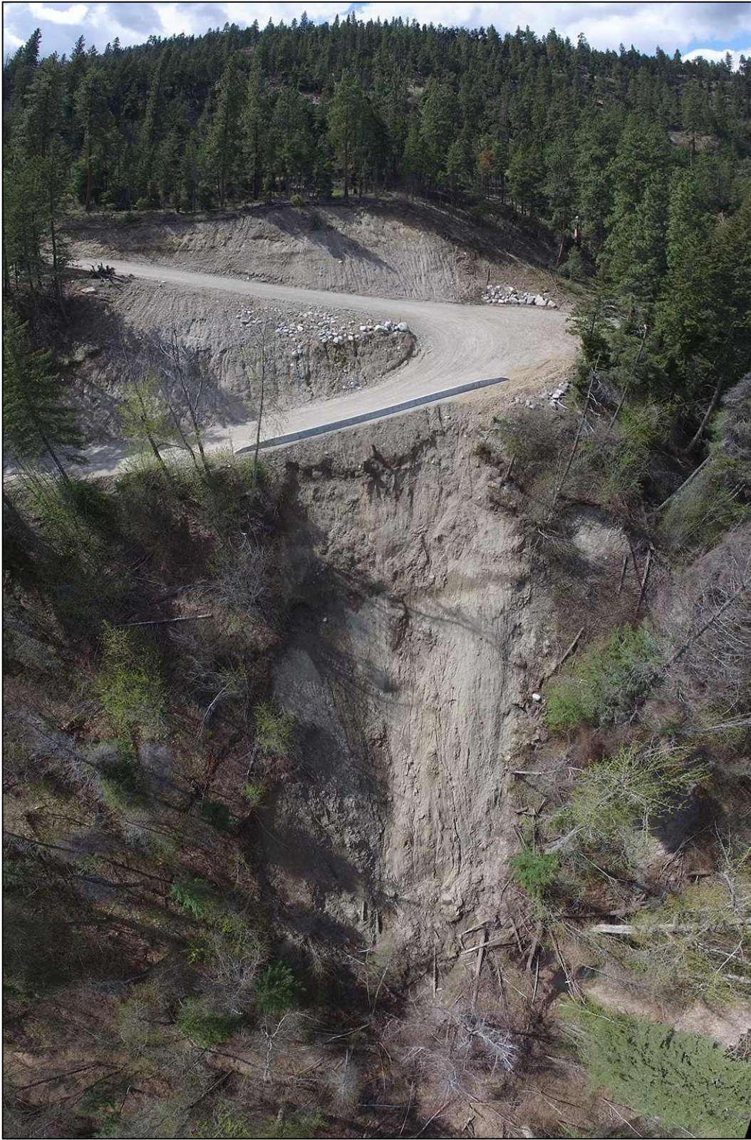
Photo stitch 6 (April 30, 2018). This landslide occurred on or about March 28, 2017. It measures about 110 feet in elevation, and about 85 feet wide at the top of the road. According to government correspondence, about 1,200 cubic meters of material fell into Peachland (Deep) Creek. The location is less than one kilometer from the District of Peachland's water intake. Turbidity readings at the intake exceeded 500 NTU as a result.
