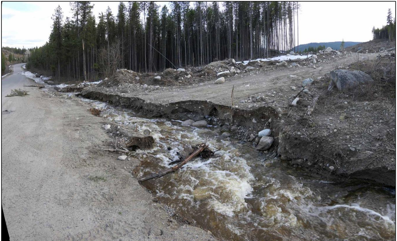
Photo stitch 71 , below (April 30, 2018). The water runoff from Photo 70 is seen heavily eroding the east side of the Princeton road, also eroding a logging access road.
