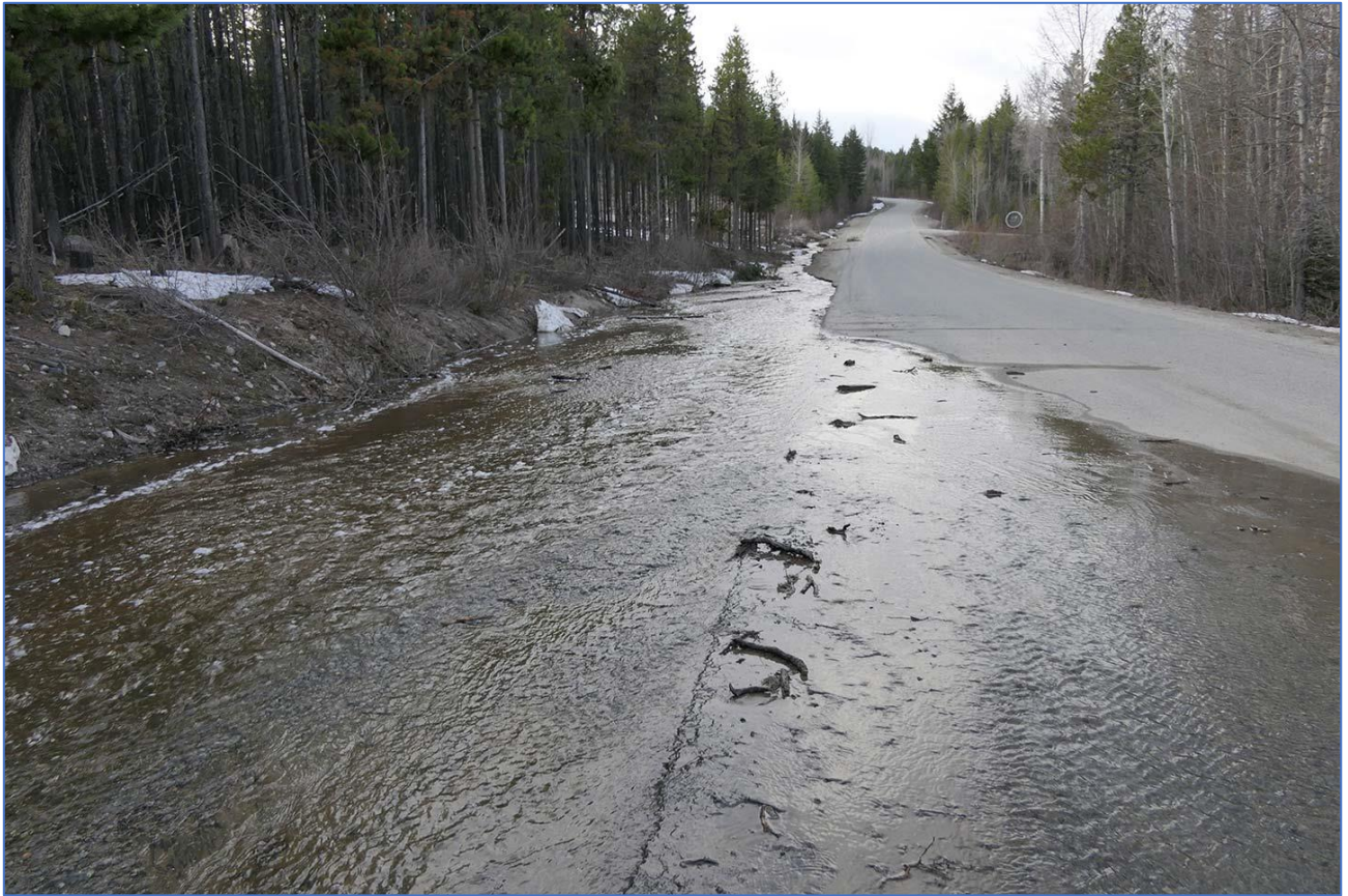
Photos 72 and 73 (April 30, 2018). About 150 meters down Princeton road from Photo 71, the raging melt water eroding the western flank of the pavement, is pouring over the road grade. Photo 73 below, reveals that the entire road was engulfed, with a wide section running over the other side of the road.
