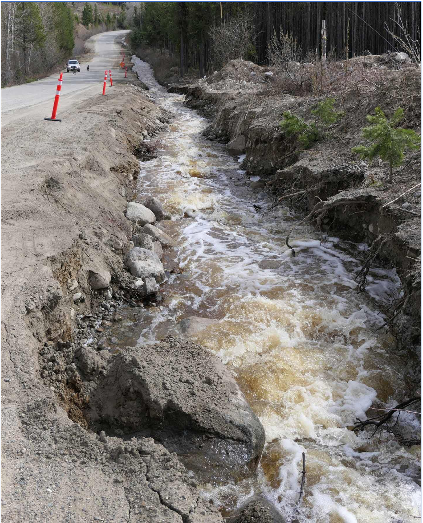
Photo stitch 74 (May 4, 2018). Four days after Photos 71-73, local highways crew have dug the Princeton road ditch here deeper, so that runoff would be contained and not spill over again.
