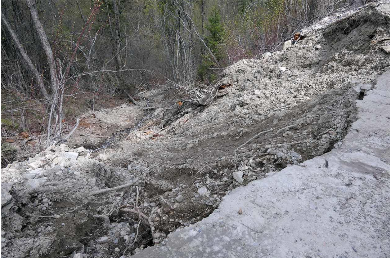
Photo stitch 16 and photo 17 (April 30, 2018). Road failure around the 3.5-kilometer mark on Munro Road. Debris has fallen into stream channel above Peachland Creek. The Princeton access road is seen in distance to left.
