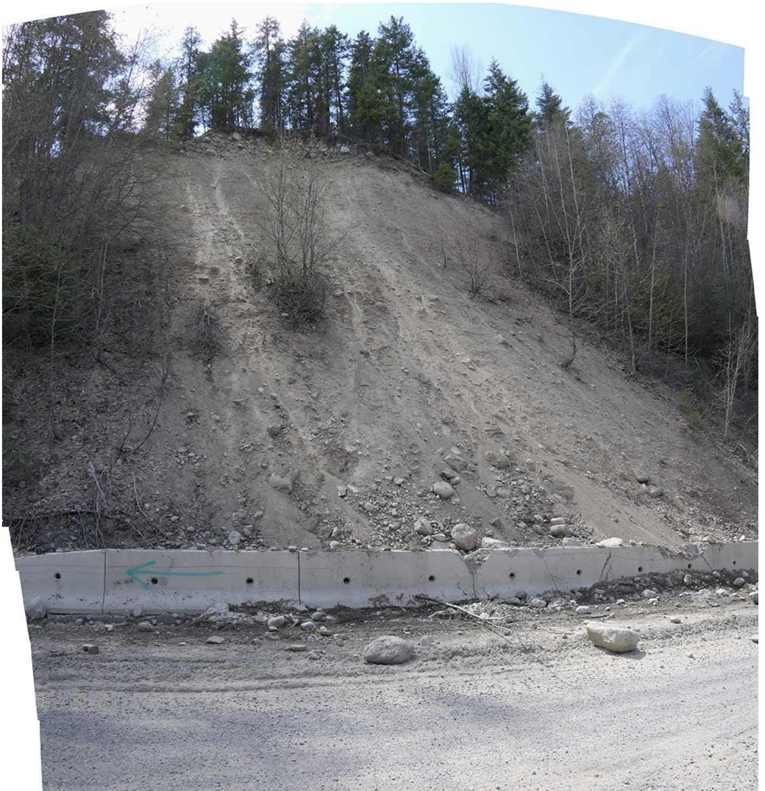
Photo stitch 23 (May 2, 2018). Ongoing steep cutslope erosion at bridge crossing over Peachland Creek, on Peachland mainline Forest Service road. Erosion of downslope or cutbank area has eroded over recent years, with silt fencing erected at bottom area beside Peachland Creek. The lower area is shown in Photo stitch 24.
