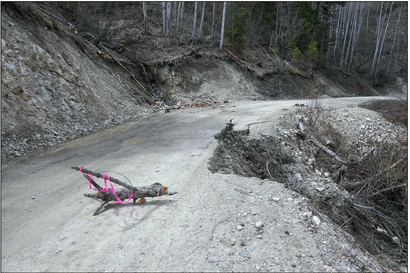
Photo 18 (April 30, 2018). Same location as photos 16 and 17, looking west and upslope. Road failure resulted from stream above road (top left), and a blocked culvert, causing wash over road.
