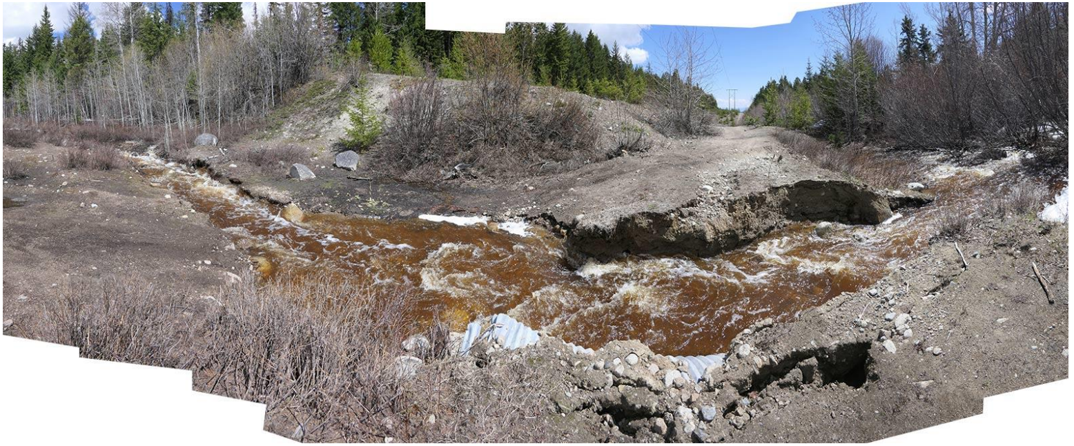
Photo stitch 64 (May 5, 2018). The increased water runoff from Wilson Lakes area is seen here cutting through BC Hydro's access road. According to a local citizen that is familiar with this area, this area began to be washed out last Spring (2017), but this year's runoff has been much greater.
