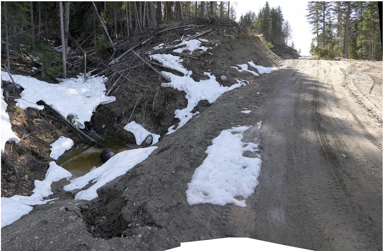
Photo stitches 36 and 37. Below, ditch water from cutslope was running strong, and eroded road prism above culvert.
