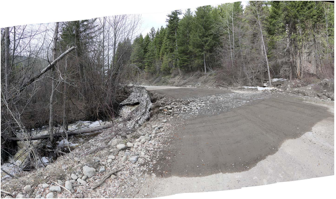
Photo stitches 44 and 45 (May 5, 2018). Small creek overflowing because the culvert is too small, and slightly plugged. Recent high water, and erosion of road prism.
