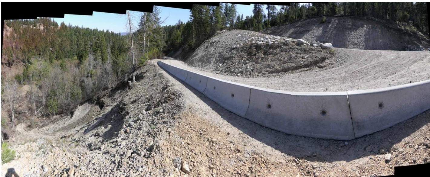
Photo Stiches 7 and 8 (April 27, 2018). Above: Looking from the top of the switchback down to the 2017 landslide. Concrete blocks were placed to protect vehicles. Below: New, and second, landslide, to the right of road, which occurred about April 22, 2018.
