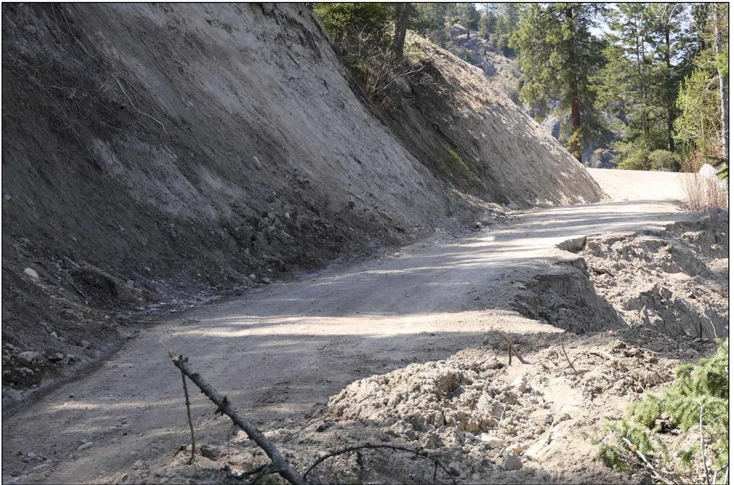
Photos 2 to 5 (April 27, 2018). Just before the first switchback, recent landslide (down to right) and collapse of glacial till and silt onto road. Signs near the area.
