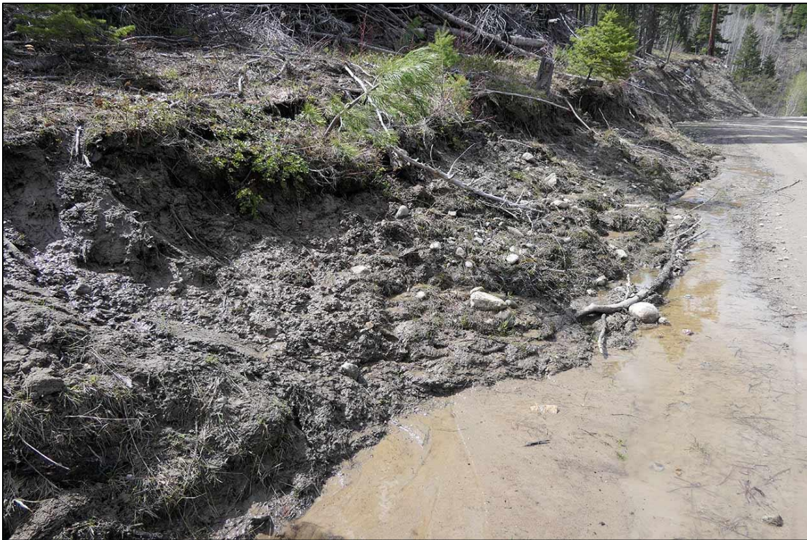
Photos 20 and 21 (April 30, 2018). Glacial silt muck oozing out of small cutslopes causing blockage of culvert and water runoff to spill across road prism and down ditches and ephemeral streams. About 4-kilometer mark.
