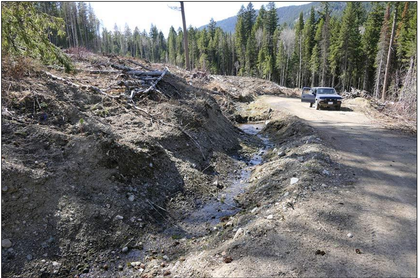
Photo 28 and Photo stitch 29 (May 2, 2018). Dominating presence of soil erosion from Spring snow melt alongside Tolko's secondary road that travels the majority of the southern flanks of the Greata Creek valley.
