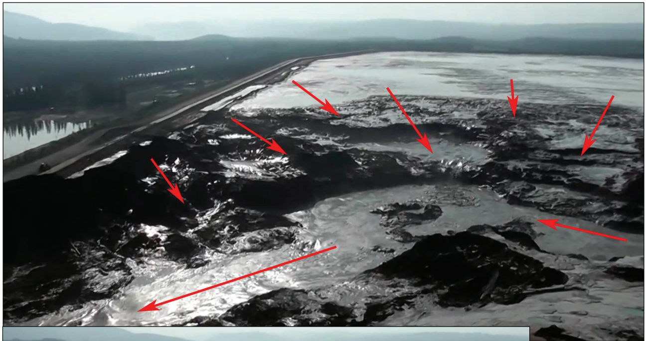
Cascading Failure Events of Saturated Tailings Mass
