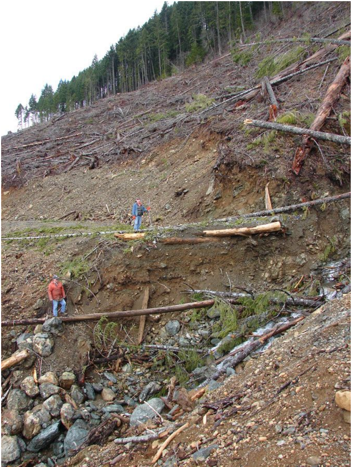
Photo 31. Showing profile of road area blowout on stream number 6, by former culvert number 27. Note the two people for scale. The road used to come across even with the person near the middle of the photo, who is standing on the road.
