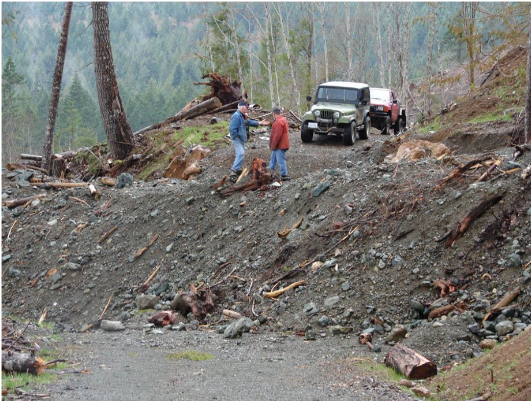
Photo 9: As far as the road goes in Block 141. Debris torrent remains some ten feet in height overtop logging road.
