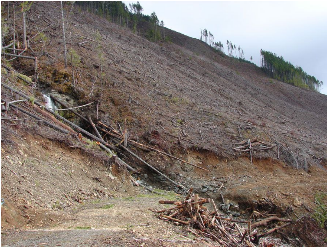
Photo 25 (above). Stream number 6 at culvert number 27. Location just below photo 24, where a dam formed, and then burst, causing a debris torrent to rush downward. Culvert was completely blown out and torn apart with the torrent.
