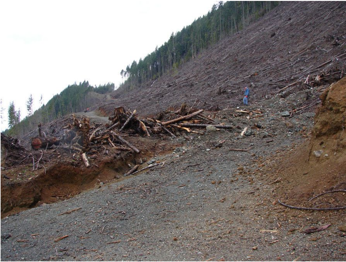
Photo 21 (above). Beginning of switchback toward upper part of stream number 6. Erosion debris of stumps, small logs, rocks and soil across road deposited from debris torrent on stream number 9 at culvert number 24. Debris height is about 8 feet or so above top level of road.
