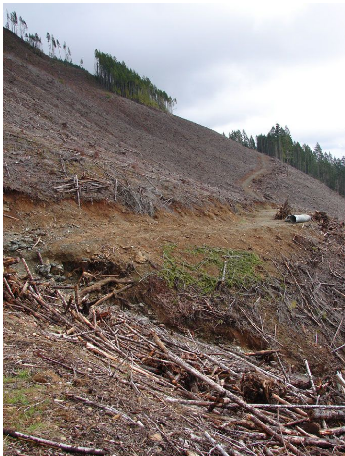
Photo 25 (above). Stream number 6 at culvert number 27. Location just below photo 24, where a dam formed, and then burst, causing a debris torrent to rush downward. Culvert was completely blown out and torn apart with the torrent.
