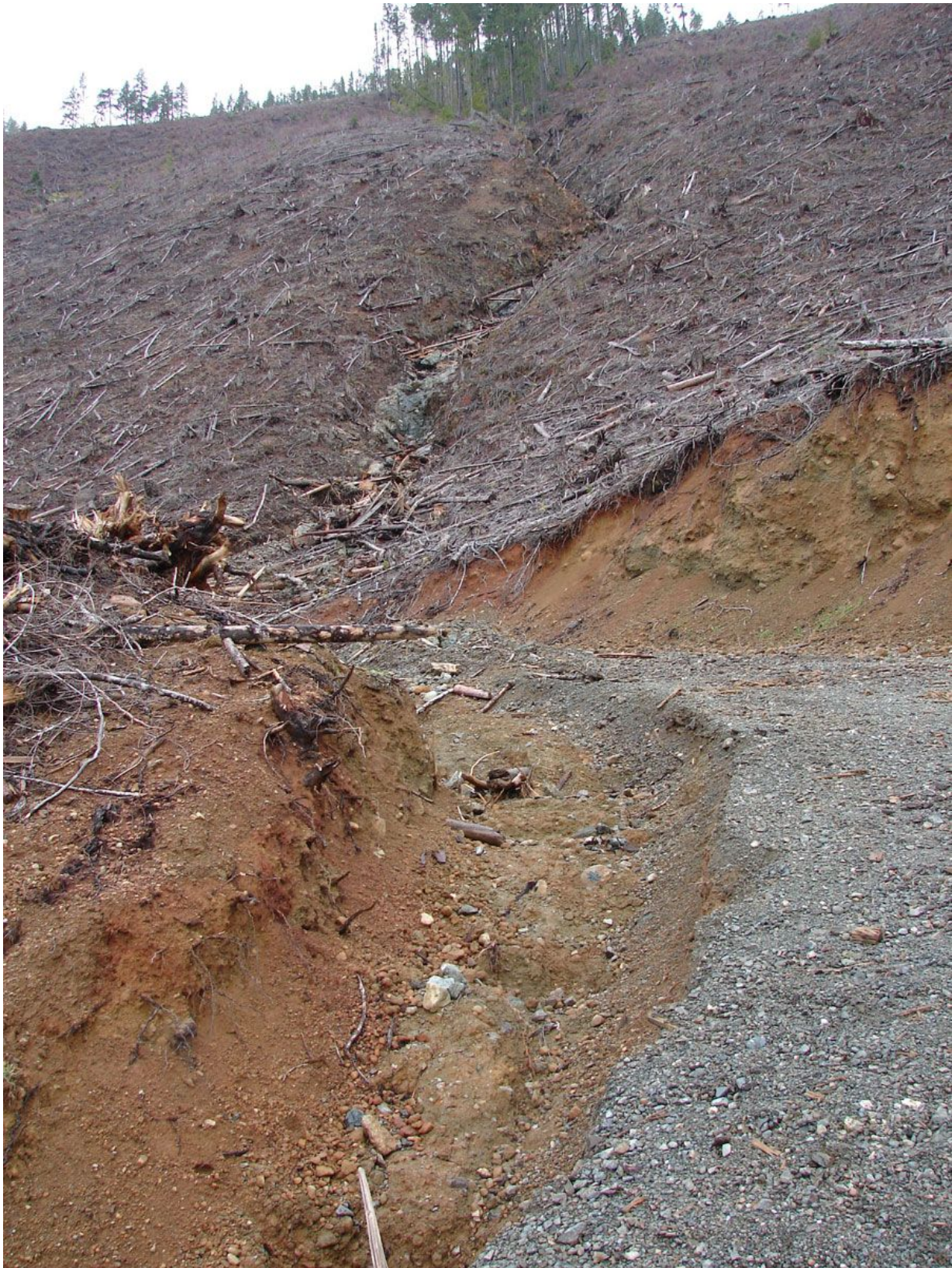
Photo 20. Diversion from stream number 9 as a result of blocked culvert (number 24), down onto the road, around corner, and over blocked culvert number 23.
