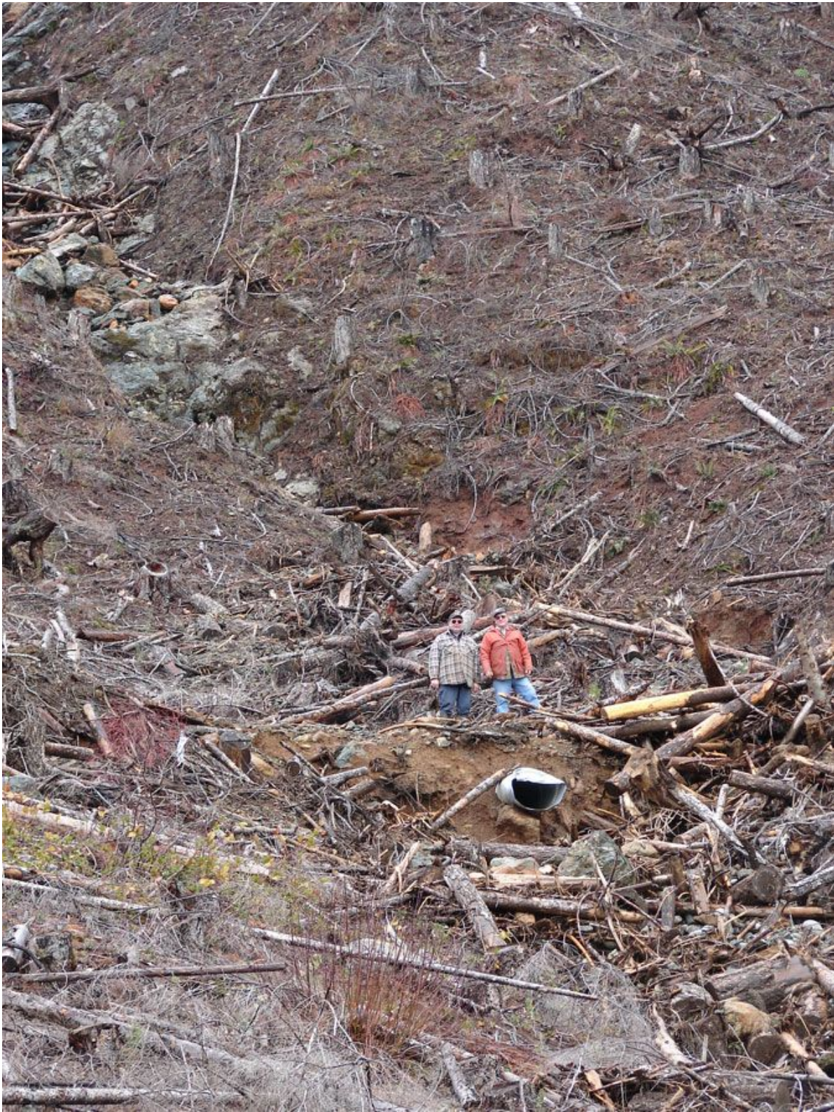
Photo 17. Plugged culvert (number 24) directly above culvert number 23 on stream number 9.
