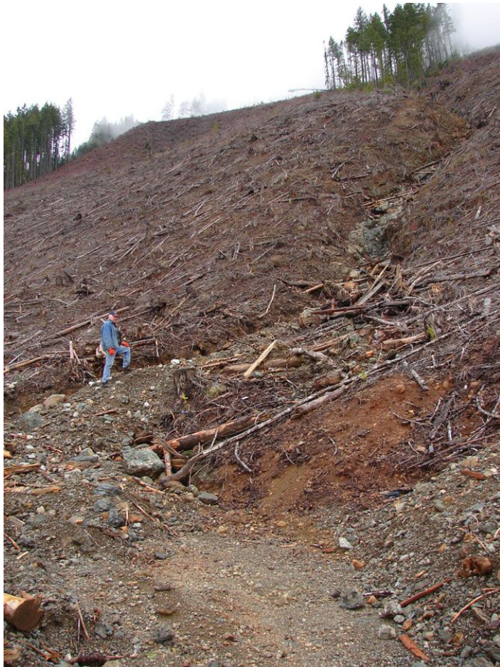
Photo 21 (above). Beginning of switchback toward upper part of stream number 6. Erosion debris of stumps, small logs, rocks and soil across road deposited from debris torrent on stream number 9 at culvert number 24. Debris height is about 8 feet or so above top level of road.
