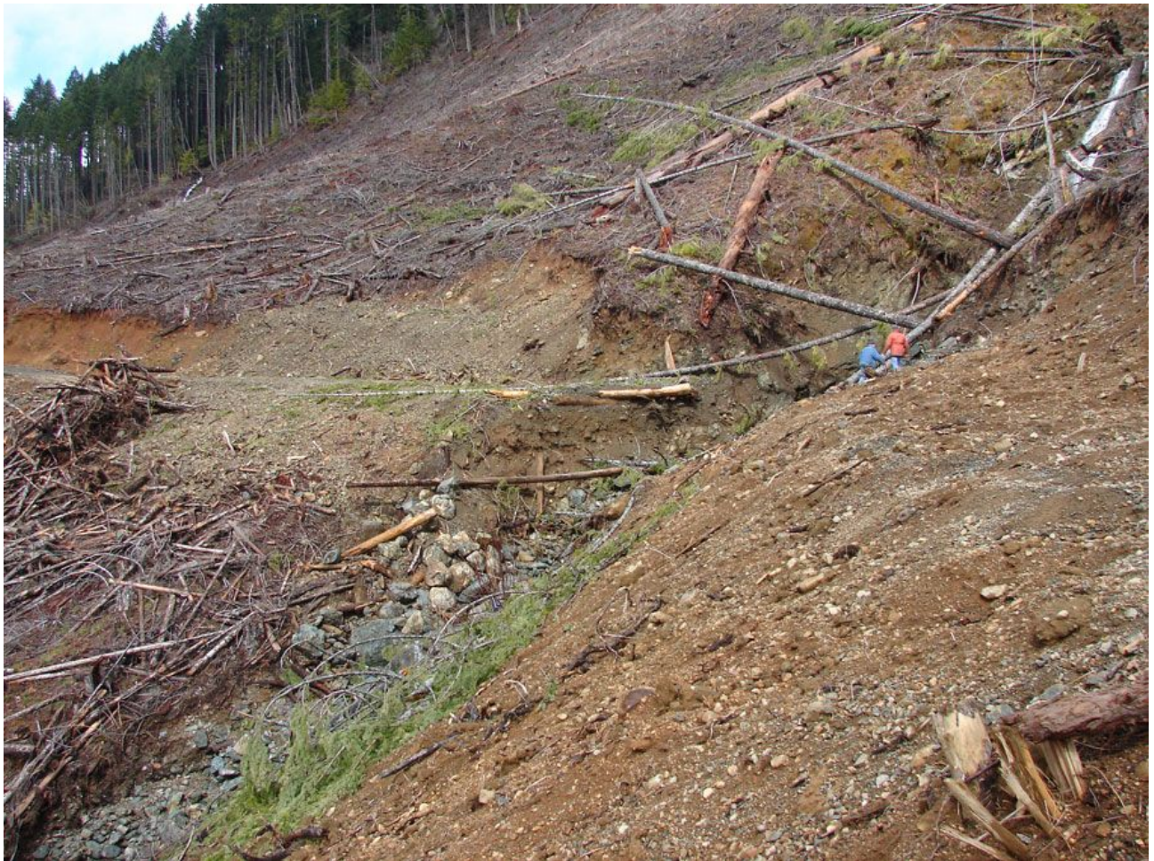
Photo 28. Looking at the blowout area on stream number 6 at former culvert number 27. Note the size perspective by two people at middle right.
