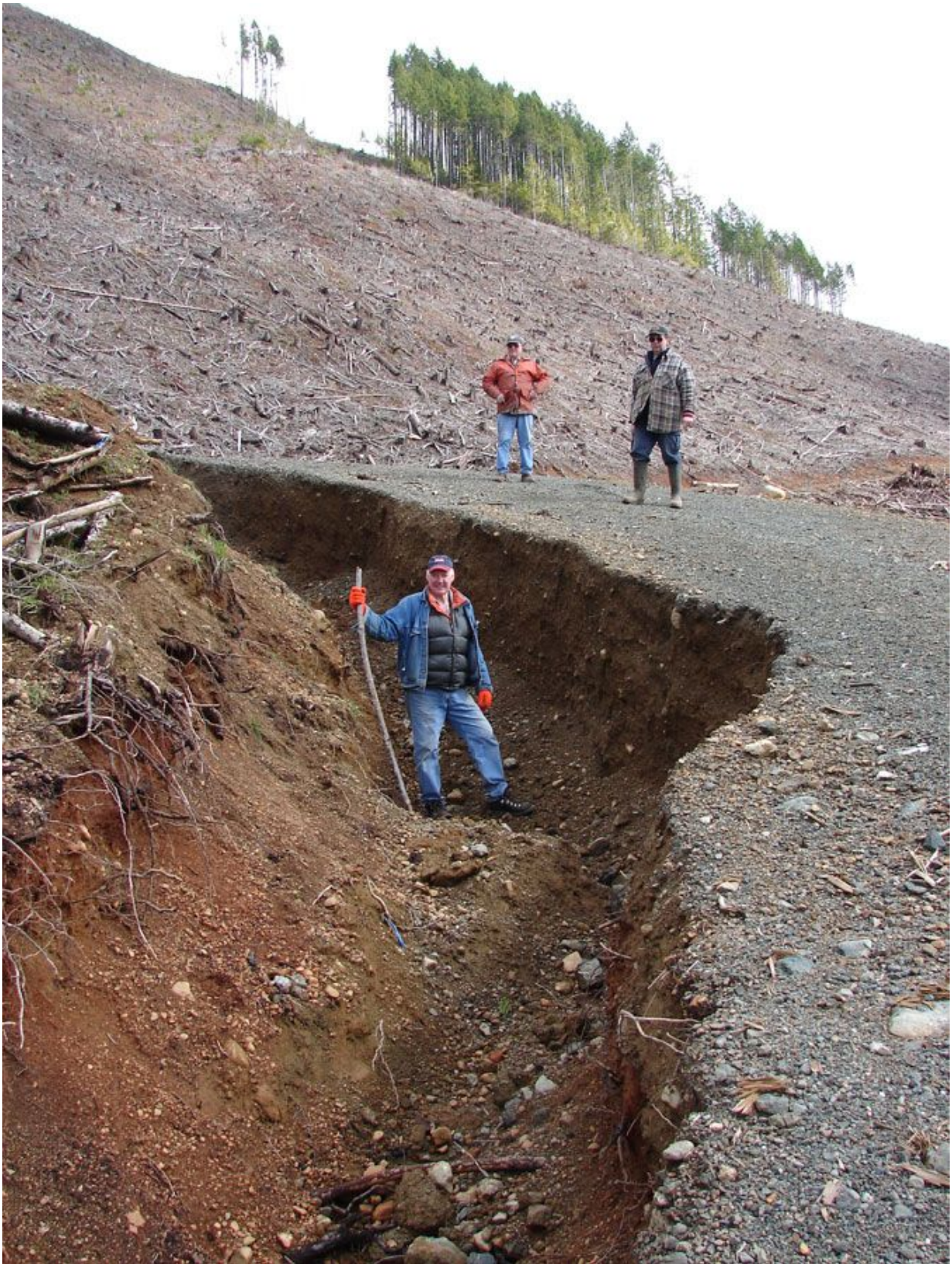
Photo 19. Extent of erosion in ditch as a result of diversion of stream number 9 above and around corner to left of photo.
