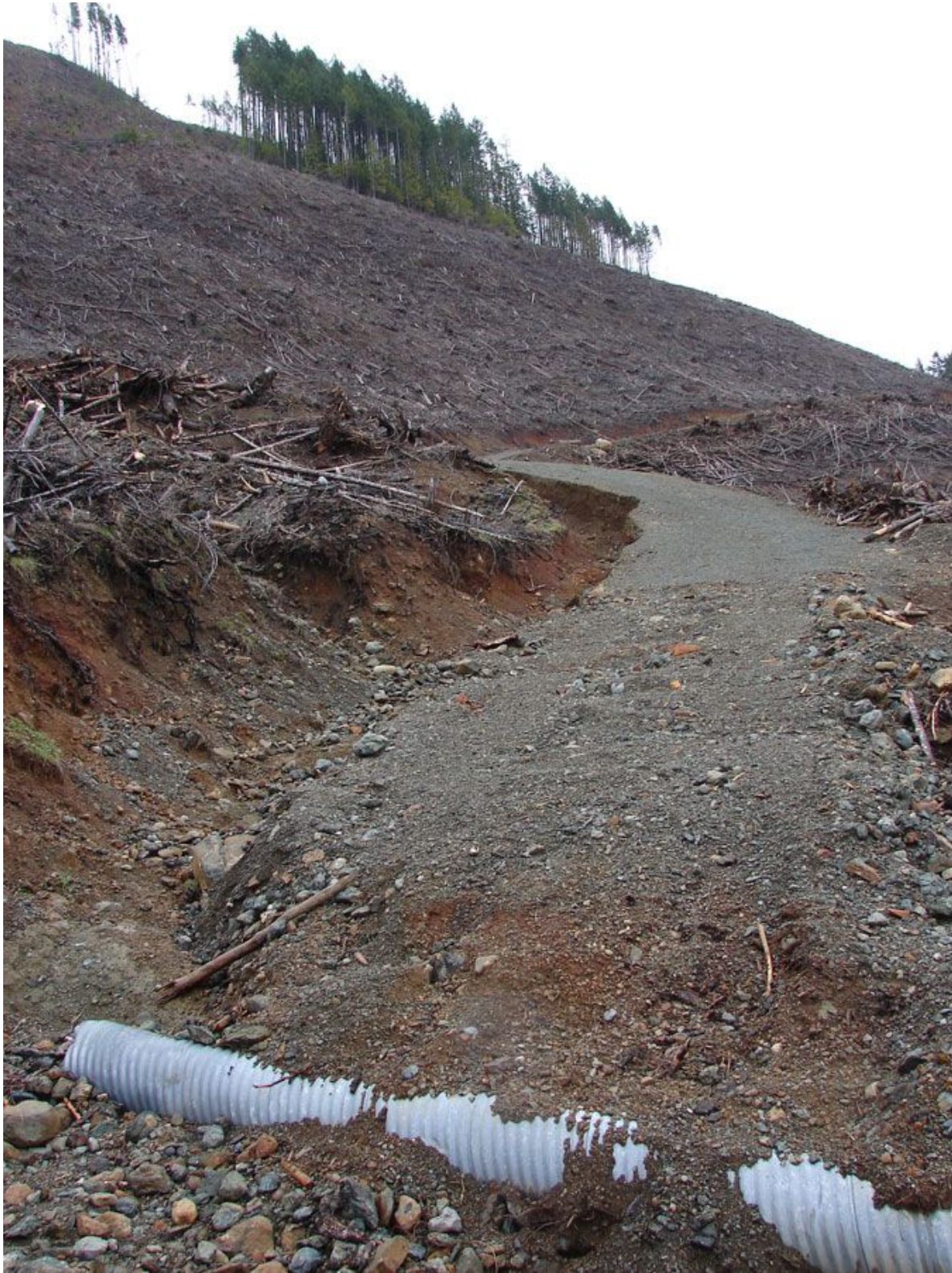
Photo 18. Looking up the road from culvert number 23 to switchback entrance (middle of photo) and ditch erosion on logging road.
