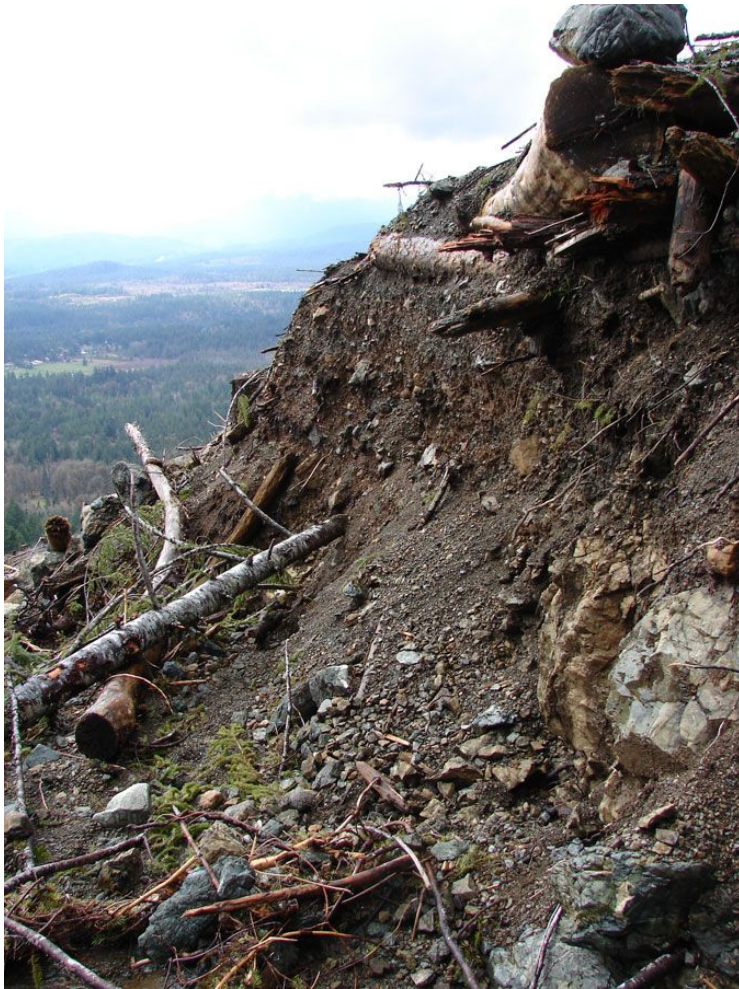
Photo 32 (left). Profile of depth of road height material remaining after the blow out on north side of road.
