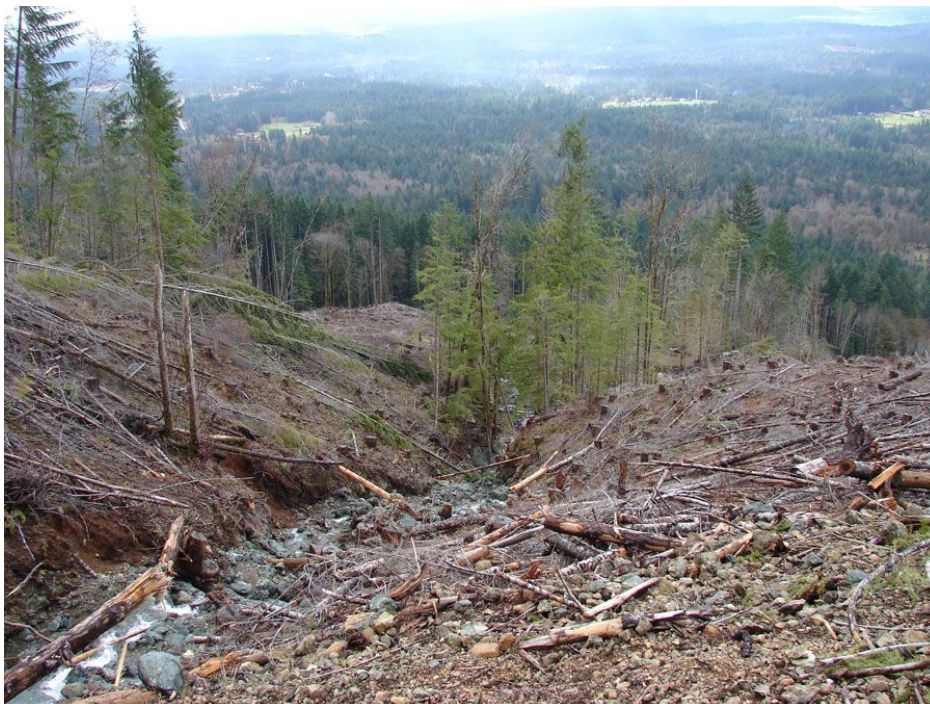
Photo 28. Looking at the blowout area on stream number 6 at former culvert number 27. Note the size perspective by two people at middle right.
