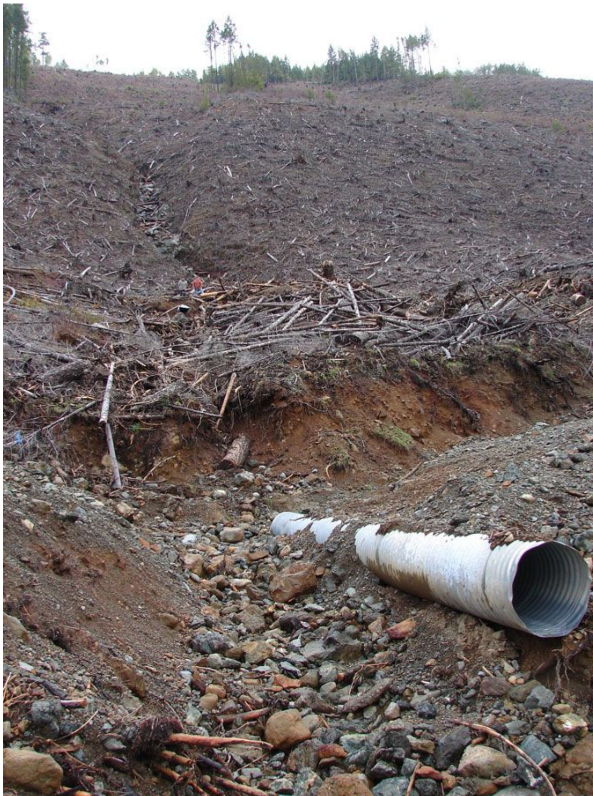
Photo 16. Dysfunctional culvert (number 23) on road along now dry bed of stream number 9.
