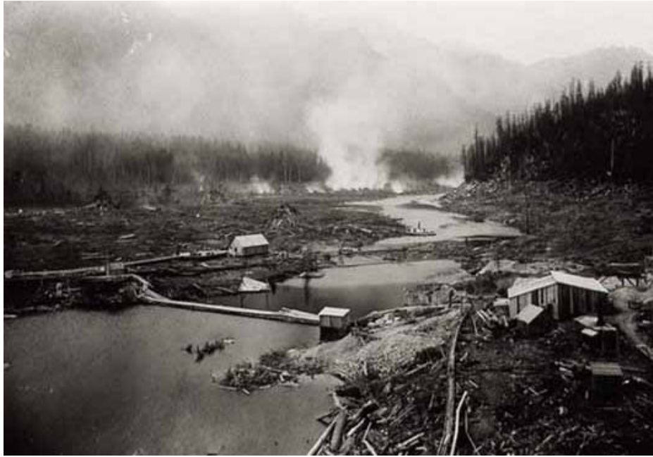
Forest clearing and pile burning operations for 70 foot flooding margin at the south end of Coquitlam Lake, around 1911. Source: B.C. Hydro archives.
