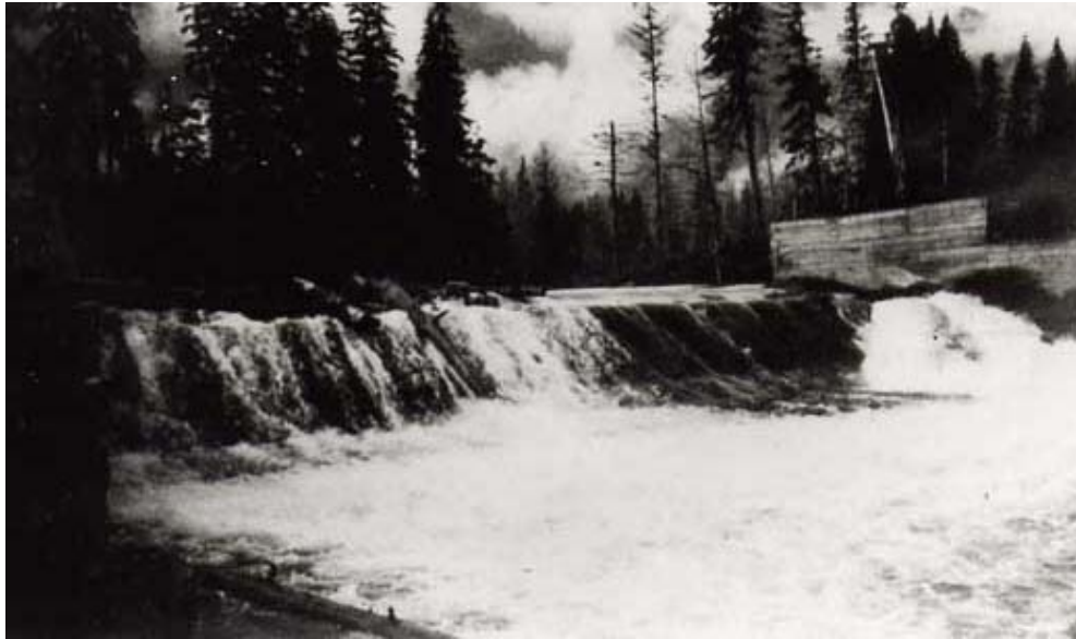
Photo of first dam, somewhere between late 1905 and 1908. Caption beneath photo reads: “Three and a half feet of water passing over the crest of Coquitlam dam.” Fish ladder on right side of dam in photo. Source: B.C. Hydro archives.
