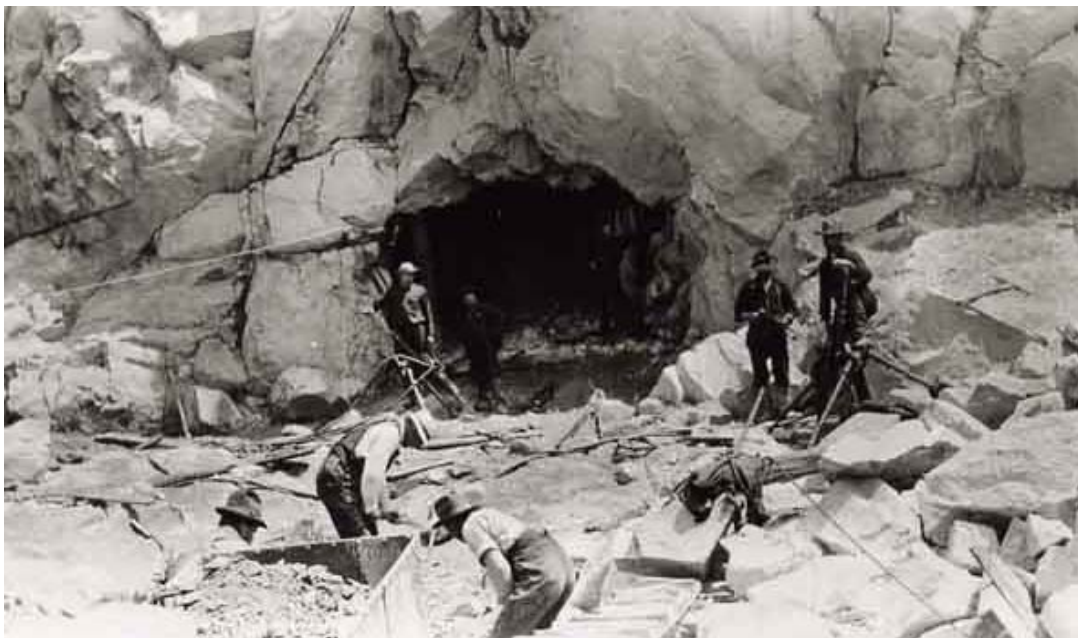
Diversion Tunnel labourers begin work for 2.4 mile excavation of granite between Coquitlam and Buntzen Lakes.
