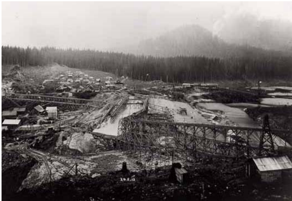
Photo taken on May 20, 1913 of the final phase of the Coquitlam dam, showing trestle bridge for sluicing and temporary construction camp with lumber mill. Source: B.C. Hydro photo archives.
