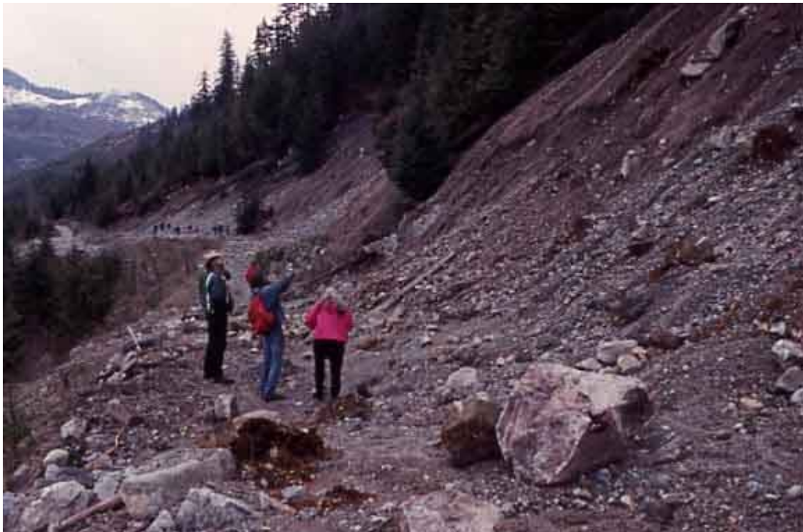
Chapman Creek, Sunshine Coast Regional District, Category 2 Watershed Reserve, May 1996. Forest previously liquidated from top to bottom. Note severe road, cutslope, upper-slope, and lower-slope erosion, landslides in distance.
