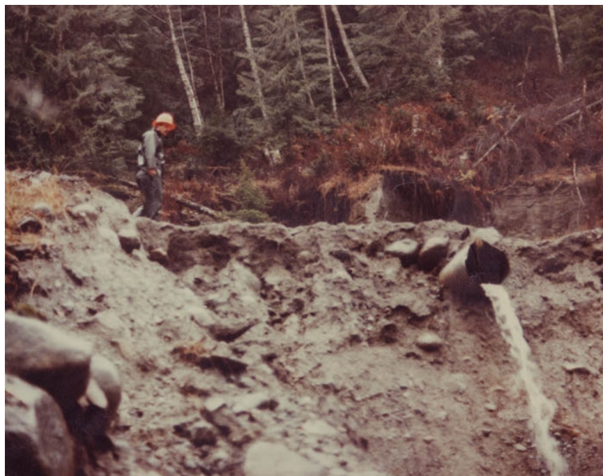
Erosion of road prism in the Capilano watershed, just above the Capilano River. Fine lacustrine silts and clays, that maintain long states of suspension (muddy water) released into the Capilano drinking reservoir.
