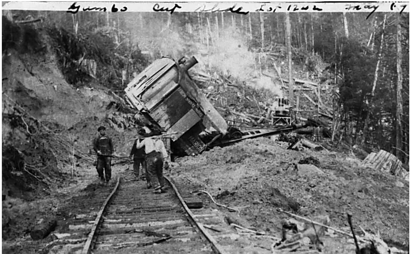
Capilano Timber Co. operations. Above: Marion steam shovel collapse under its own weight in muck. Below: Exposed silt bank in preparation for railway track. Many operations were ruining water quality.
