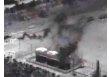
Invisible gas leakage (made visible) from gas storage tanks at a drilling site in Texas.
