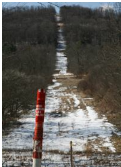
An underground gas line in Dimock, Pa. (Abraham Lustgarten/ProPublica)
