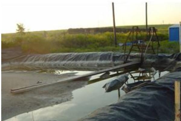
This photo, taken Oct. 5, 2007, is of the underground injection disposal well site outside Fort Worth, Texas, that had passed the Railroad Commission's inspection on Sept. 27, 2007. On their second visit two months later, inspectors found several violations, including dikes that did not meet the facility's holding capacity. (Photo courtesy of Sharon Wilson)
