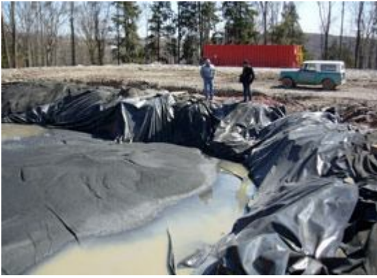
An open well pit in Susquehanna County, Pa., holds the sediment from a freshly-drilled well. (Credit: Edward Marritz)
